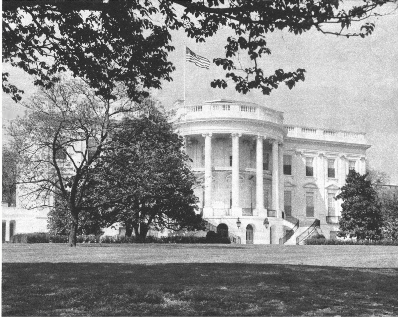
IKE AND MAMIE'S NEW HOME: The White House, a $40,000,000 mansion with no front door
